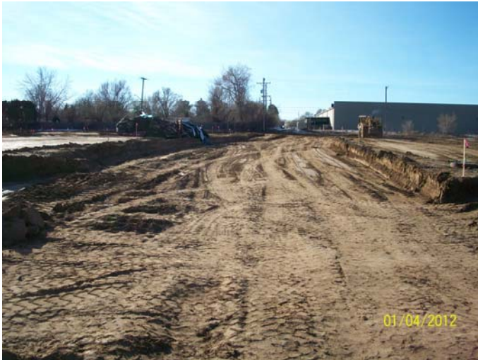
Vance Street road grading.
