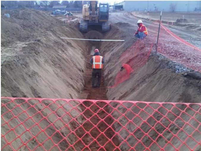
Vance Street water line trench and installation.
