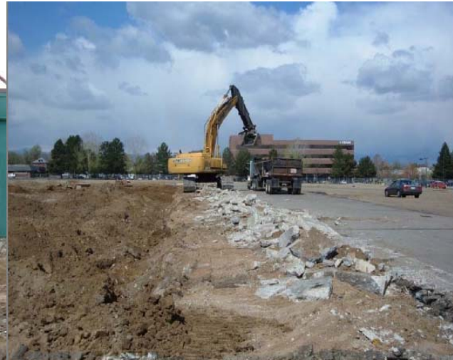
Loading trucks with north building footings for recycling.
