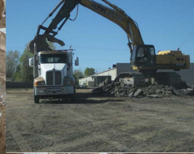
Loading asphalt to haul for recycling.
