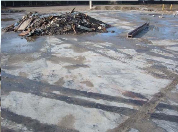
Antique Mall slab with tile removed and stockpiled for disposal.
