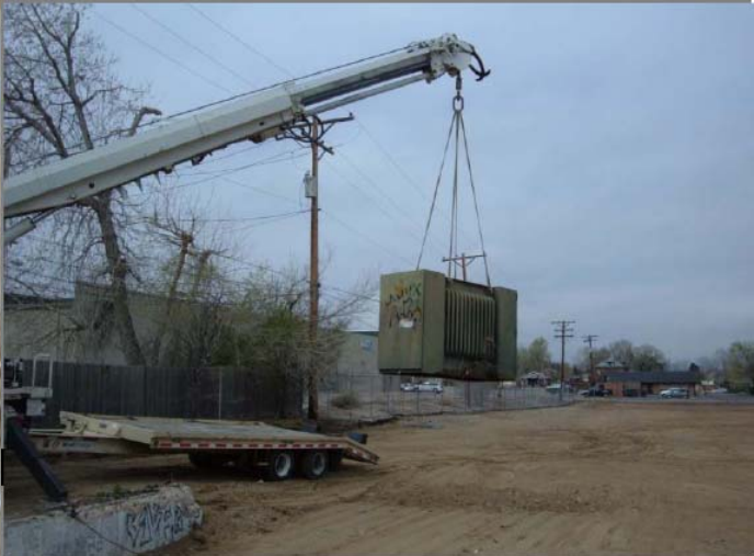
Xcel Energy removing ground transformer from site.
