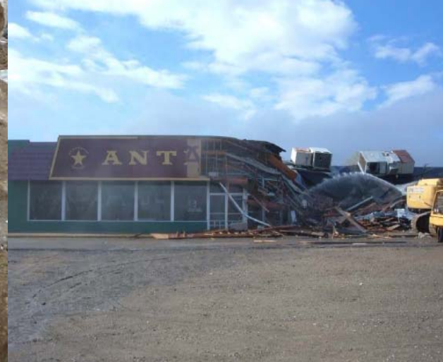
Demolition activities at former antique mall.
