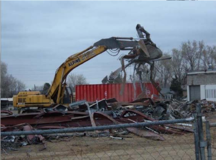
Loading out scrap metal for recycling on west portion of Antique Mall building.
